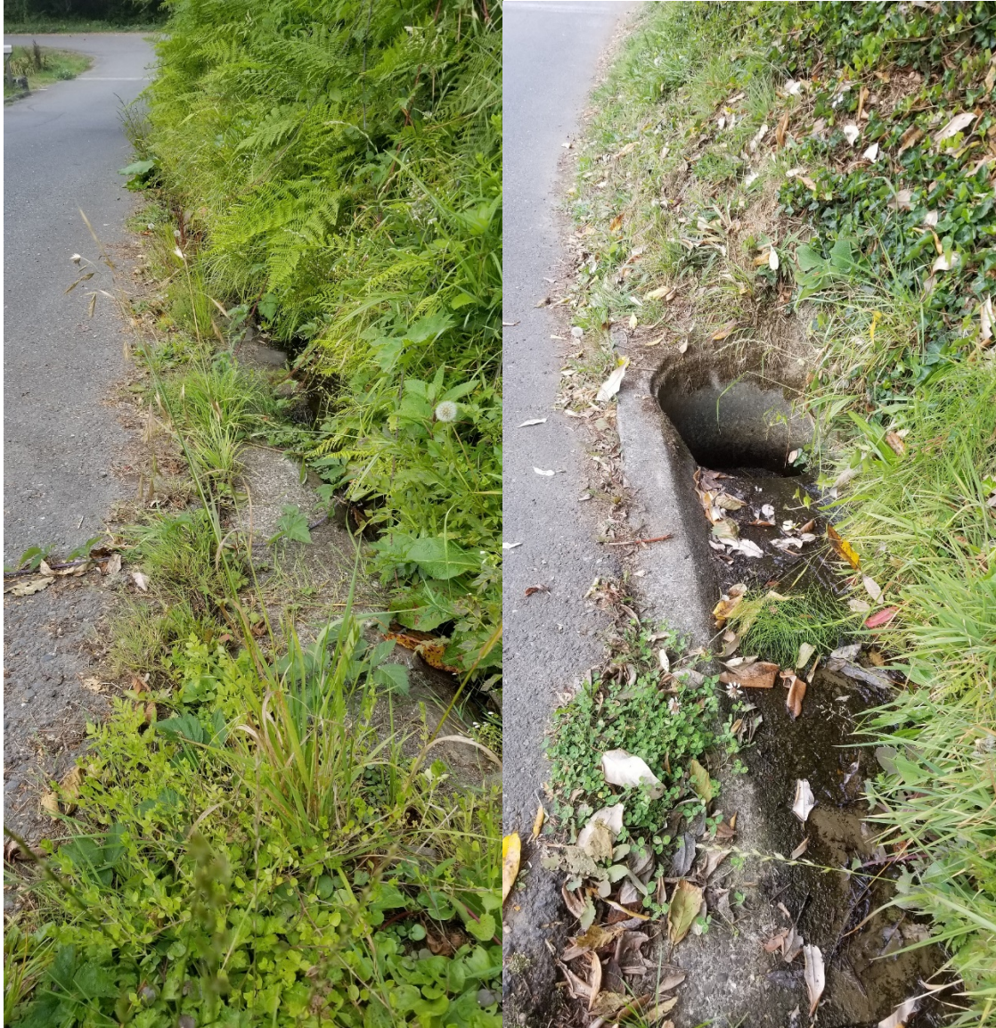
Vegetation leading up to drop inlet and culvert near the entrance of Patrick Creek Drive. Abundant vegetation along the drainage ditch may interrupt the flow of water.
