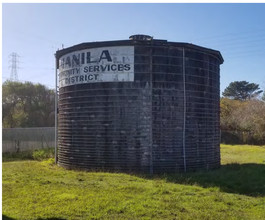
Figure 3: Existing Redwood Storage Tank
